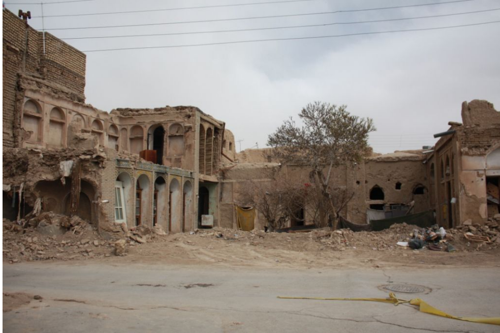
Fig.5. Some destroyed places by the lanes (Masjid Jame district)
