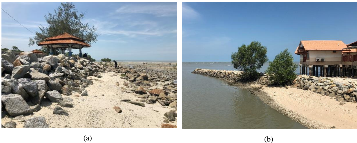
Figure 11. Current condition showing the construction of wave breakers at (a) Pantai Bagan Nakhoda Omar; and (b) Dorani Bayu Resort
