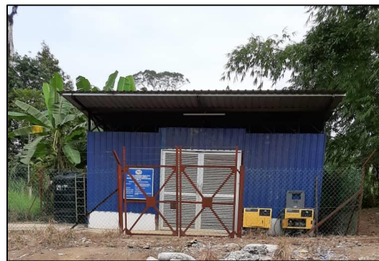
Figure 13. Existing water pump house at Kampung Gob
