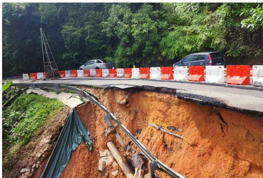
Figure 2. Slope failure at FT006 section 46.80 at Balik Pulau
