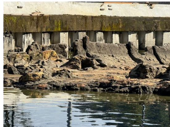
Figure 8: The Malin Kundang monument at Pantai Air Manis, Padang, viewed at low tide; current surface condition. (Source: Field work 2025)
